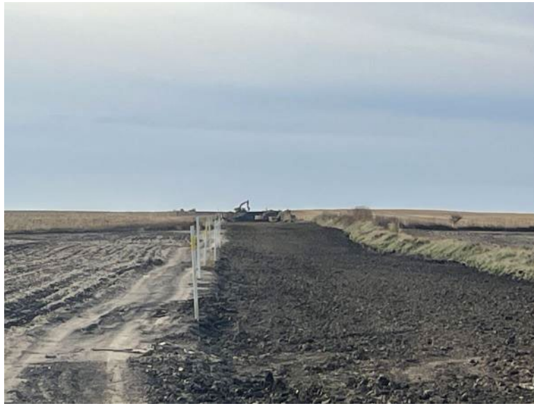
Facing south at MP 33.8, K&K restoring topsoil south of 165th Street
