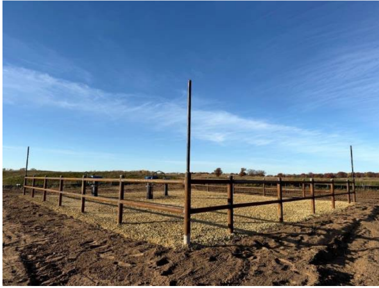
Facing southwest at MP 1.90, Farmington tie-over valve setting completed
