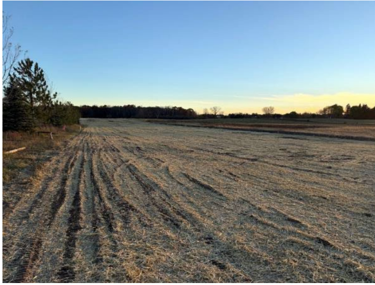
Facing south near MP 0.01, temporary workspace is seeded, mulched, and crimped
