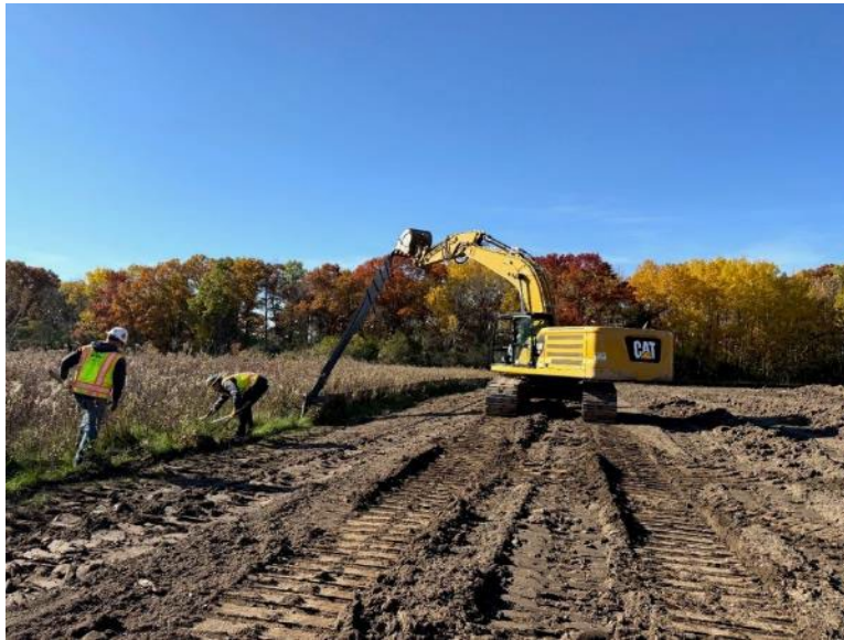
Facing west near MP 0.57, contractor removing the silt fence for final restoration
