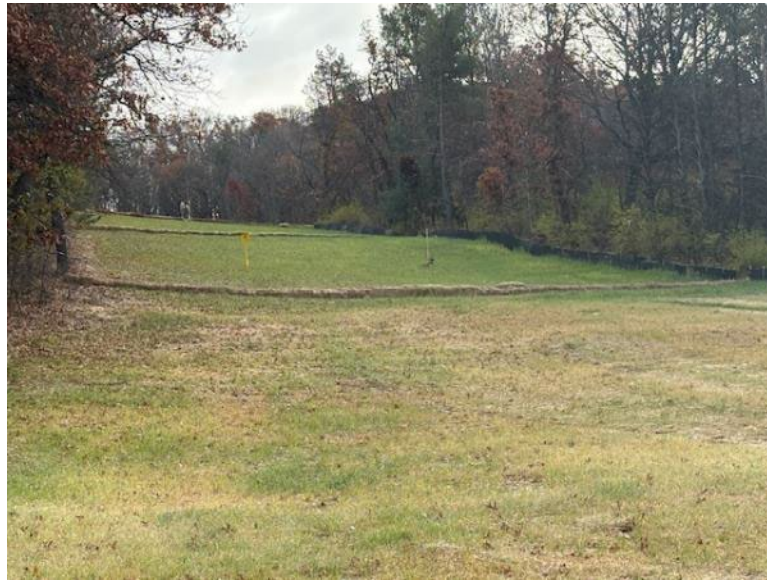
Facing east near MP 2.25, slope breakers are functional, and area is revegetating
