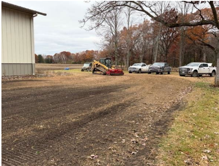
Facing east near MP 0.55, contractor drill seeding the temporary workspace and access road
