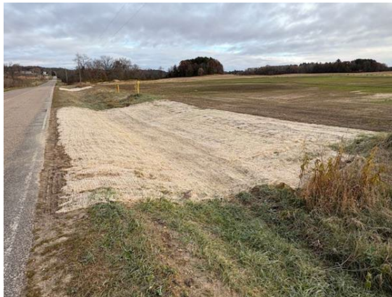
Facing north near MP 3.55, erosion control blanket (ECB) functional and staging area restored with cover crop emerging
