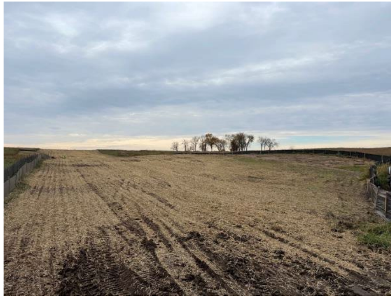
Facing south near MP1.34, temporary workspace seeded, mulched, and crimped
