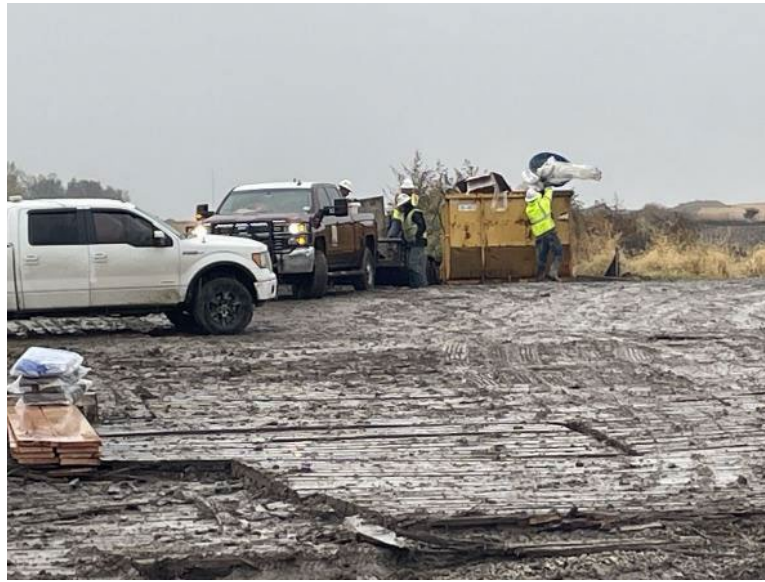
Facing south at MP 34.19, K&K loading dumpster with construction debris for removal
