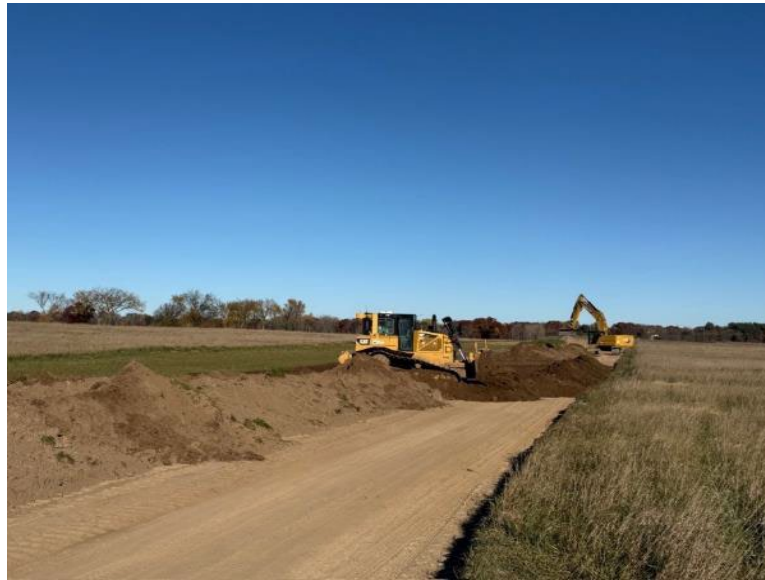
Facing north near MP 1.60, contractor restoring travel lane topsoil
