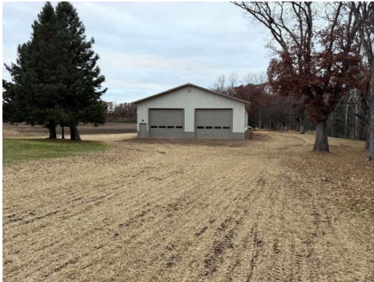
Facing west near MP 0.55, temporary workspace seeded, mulched, and crimped
