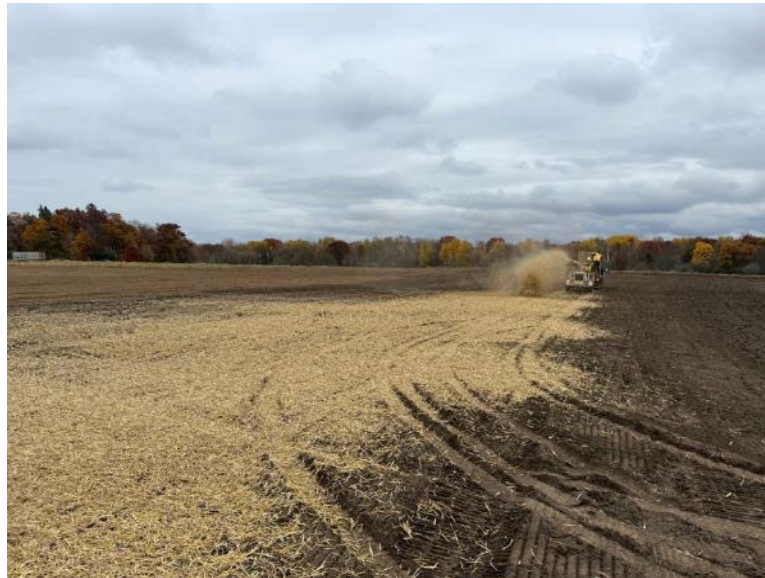
Facing south near MP 0.05, contractor mulching the temporary workspace with certified weed free straw
