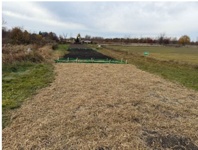
Facing west, remediation completed at HDD P4-5 exit side
