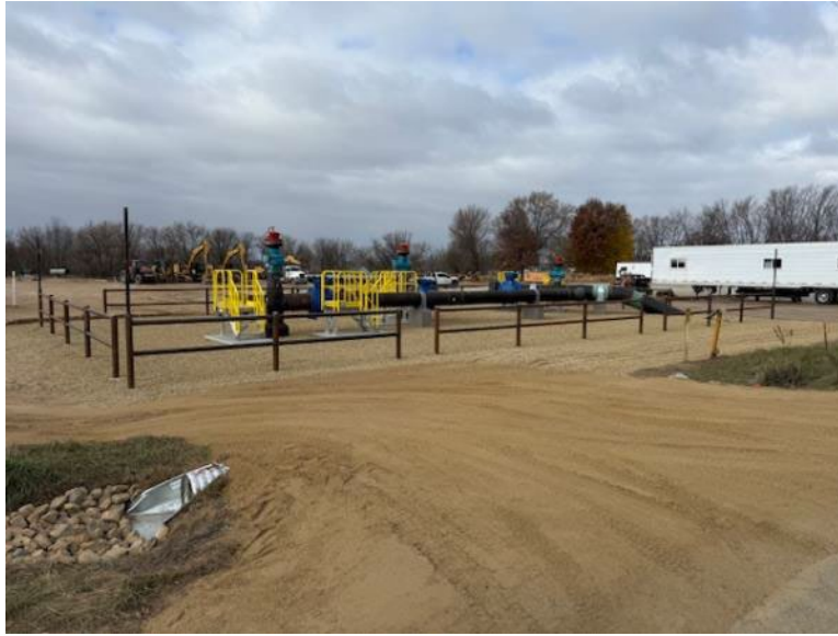
Facing west near MP 3.42, at the Elk River tie-over
