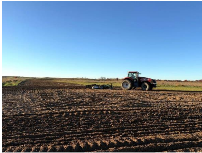
Facing south near MP 1.75, contractor discing the upland area prior to temporary seeding
