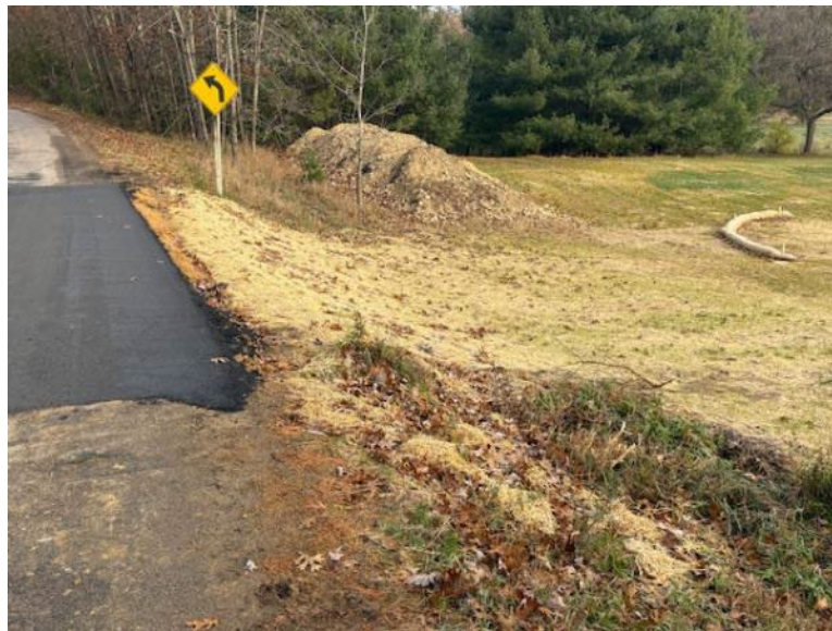
Facing north near MP 2.55, erosion controls are functional, and area is revegetating
