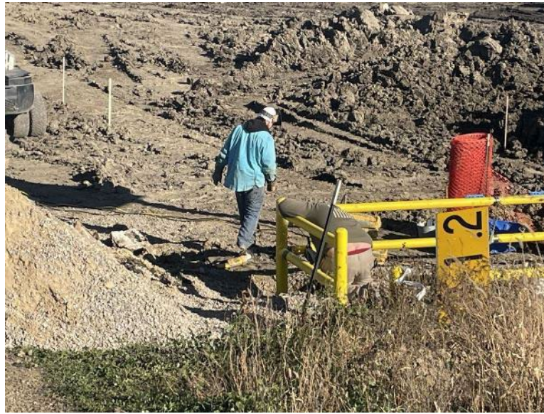
Facing north at MP 31.2, K&K welding bull pen around farm tap north of County Road 9/135th Street
