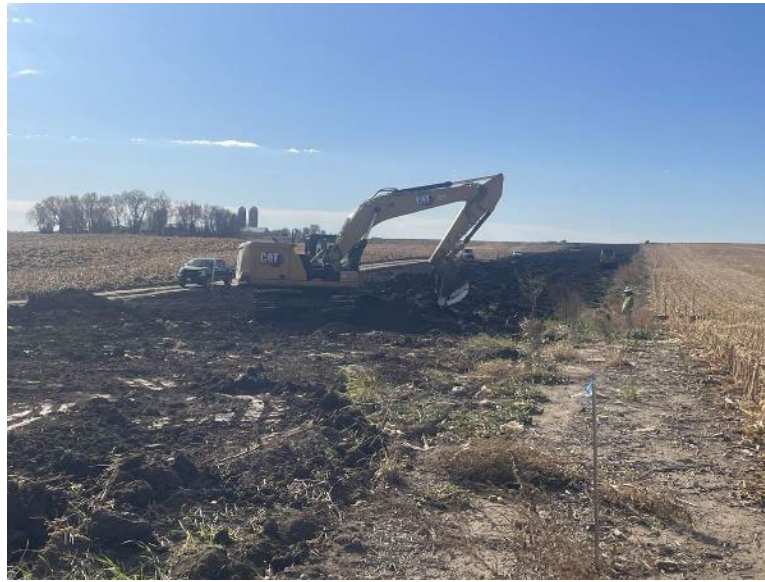
Facing southeast at MP 34.2, K&K restoring topsoil south of 165th Street
