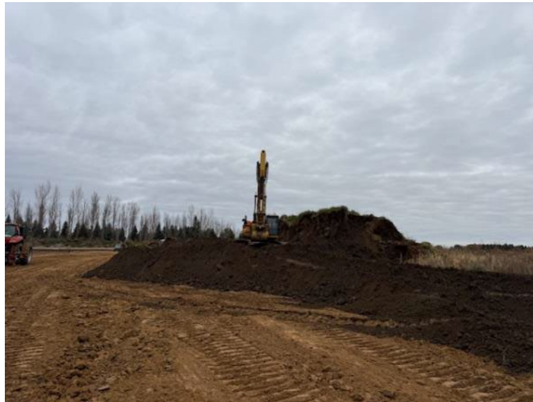
Facing north near MP 3.24, restoration ongoing
