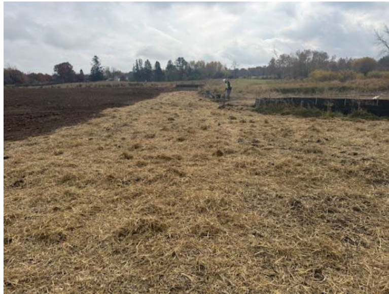
Facing south near MP 1.36, restoration ongoing
