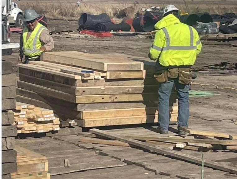
Facing north at MP 34.2, K&K constructing forms for thrust blocks
