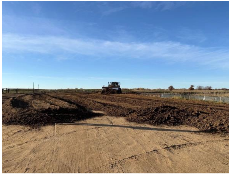
Facing west near MP 1.90, contractor grading topsoil
