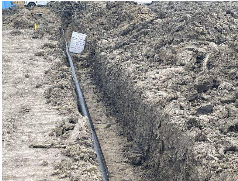
Facing east at MP 31.22, completed drain tile repair north of County Road 9/135th Street
