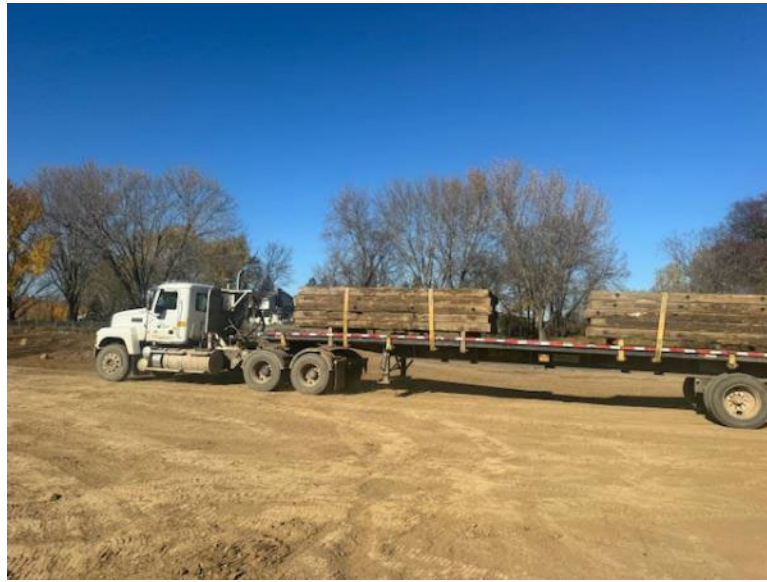
Facing south near MP 3.30, clean-up ongoing
