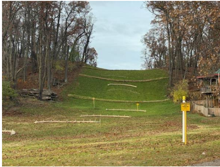
Facing west near MP 2.51, slope breakers and straw wattles are in good condition and slope is revegetating
