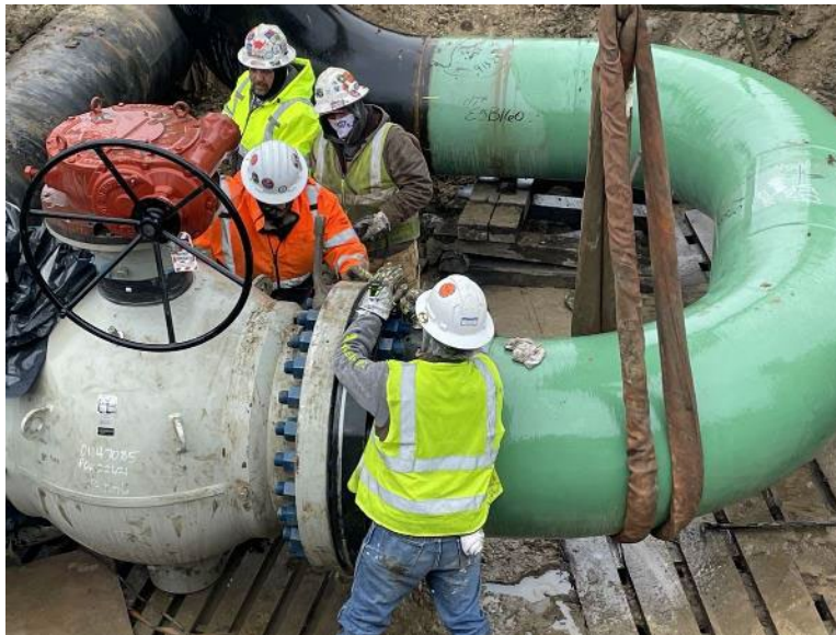
Facing north at MP 34.2, K&K torquing D-line tie-over flange bolts
