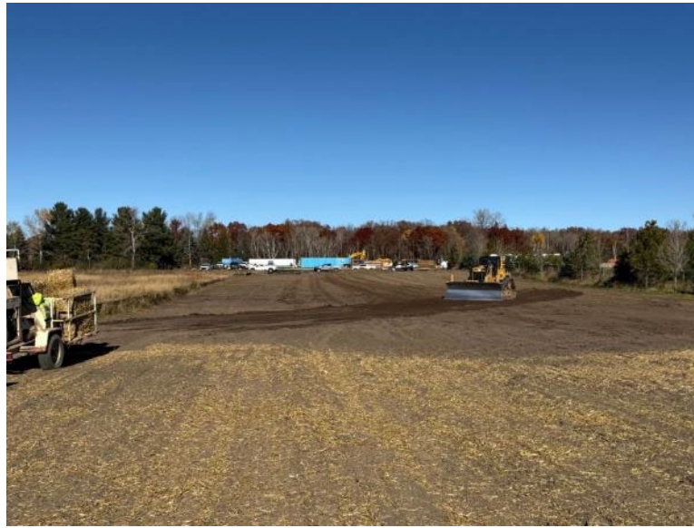
Facing north near MP 0.1, contractor continuing restoration
