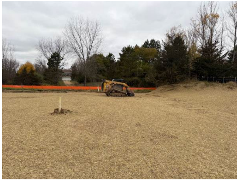
Facing west near MP 1.00, winter stabilization in progress on disturbed areas
