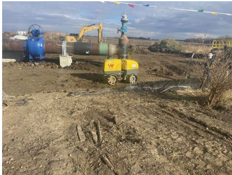
Facing north at MP 34.2, K&K compacting backfill around D-line tie-over piping
